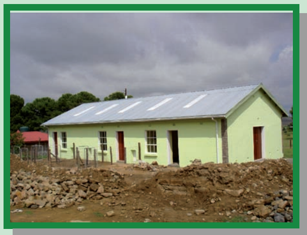
Completed shearing shed
